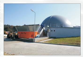
To keep the allowable concentration of H2S in biogas at appliance inlet valves, a desulphurization device is installed, working on the principle of H2S oxidation with sulphur bacteria in aqueous environment to produce elementary sulphur.
