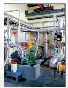
The digestion tank machine room houses pumps for sludge heating through a heat-exchanger and pumps used to transfer the content of stage I digestion tank into the stage II one.
