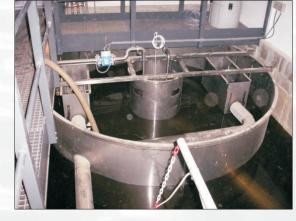
treatment process. Aerobic-stabilized sludge is pumped from the sump bottom and transported with faecal trucks for dewatering in a bigger waste water treatment plant. Iron sulphate Fe2(SO4)3 can be dosed into the sludge separation stage or downstream denitrification (into the distribution facility of the biological stage).
